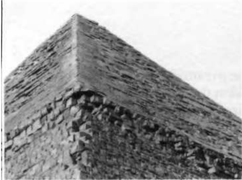
Casing blocks still intact at top of Chephren pyramid give a notion of the appearance of the pyramids prior to their being pillaged of their casings.
